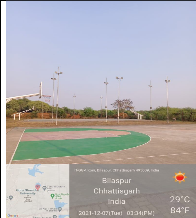
LED flood light in university Sports arena
